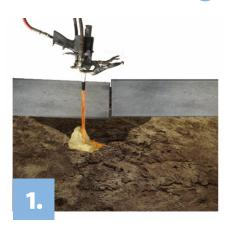
Polyurethane is injected into the void through the slab.
