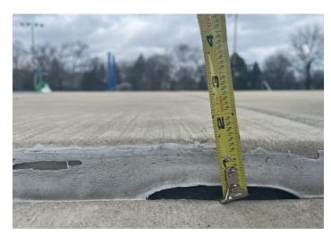
ABOVE: An example of a 1.5 inch lip created by a section of pool deck settling.
